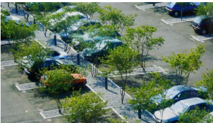
Tree planting and low-impact development integrated in parking lot islands
