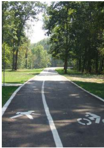
Trails with dedicated space for cyclists and pedestrians should be a minimum 4.5 metres wide
